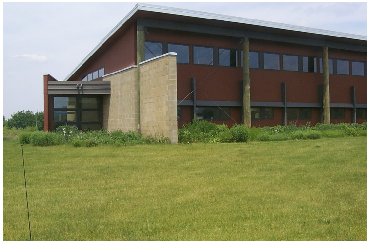
Figure 3.5. Southwest corner of the IAMU's north wing. Notice the many exterior shading devices. (John Burnet, IAUM)
