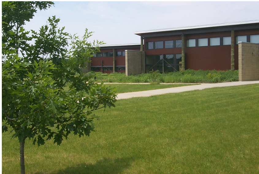
Figure 3.1. The south side of the IAMU facility; the south wing is in the right side of the picture and the north wing is in the left side of the picture. (John Burnet, IAMU)
