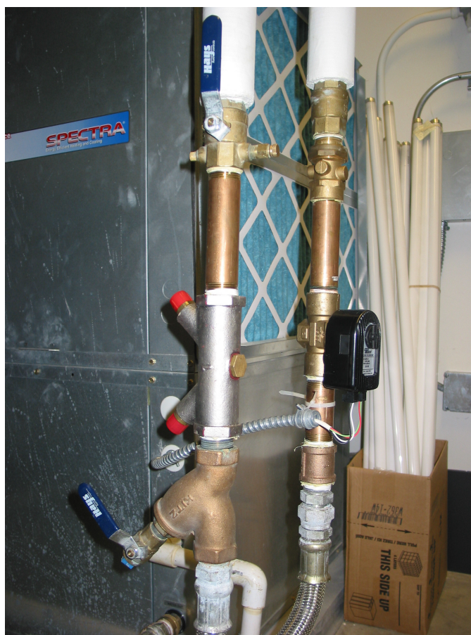
Figure 5.11. New heat pump connection piping configuration.
